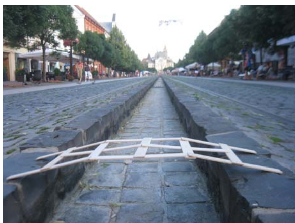
Figure 3. A 60-cm Leonardo bridge assembled in downtown Kosice
