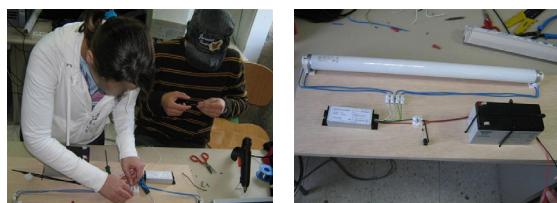
Figure 15. Fluorescent lamp with 12V ballast and lead-acid battery
