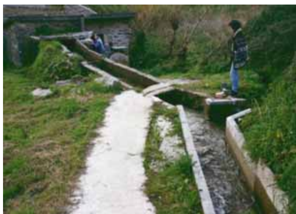
Figure 2. Mill and water channel (lead)
