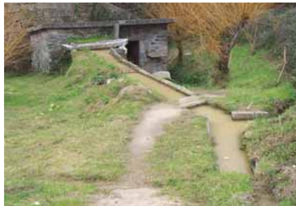
Figure 6. Mill and water channel (levada)
