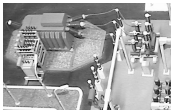
Figure 8. Close-up on main transformer (left) and circuit breakers (right)
