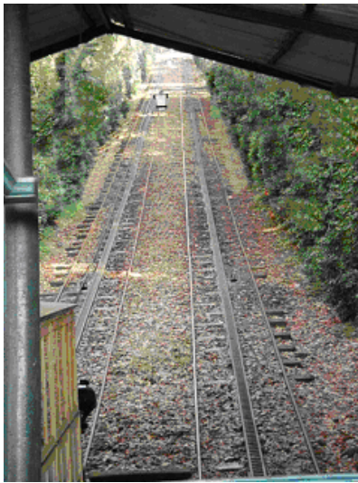
Fig. 3. The “Elevador do Bom Jesus”: the tracks
