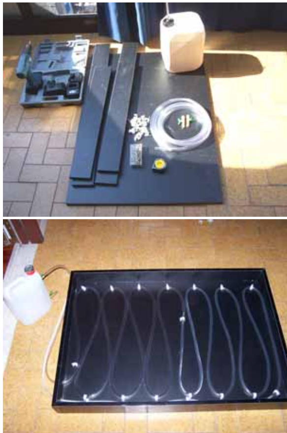
Photos 2 and 3: The preparation and construction of a serpentine solar water heater (Scuola Secondaria di 1° Grado C.B. Cavour, IT)
